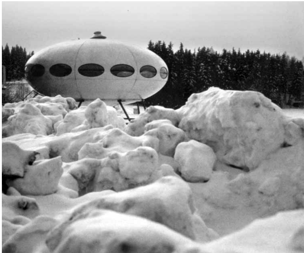
Dům Futuro. Foto z knihy Futuro. Tomorrow's House from Yesterday, 2002
